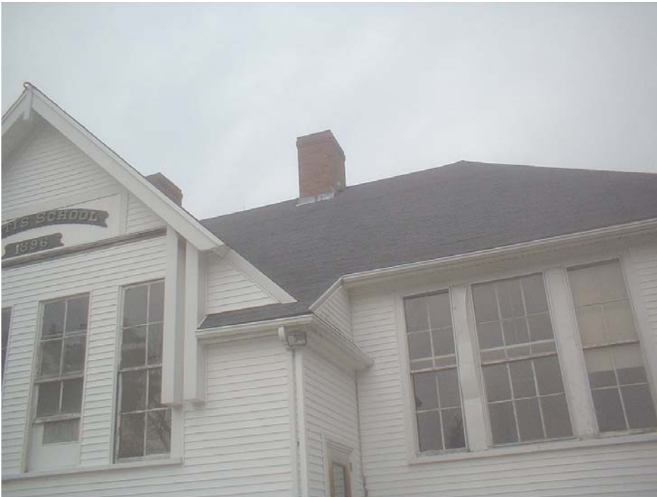
Exterior detail view of roof condition.
