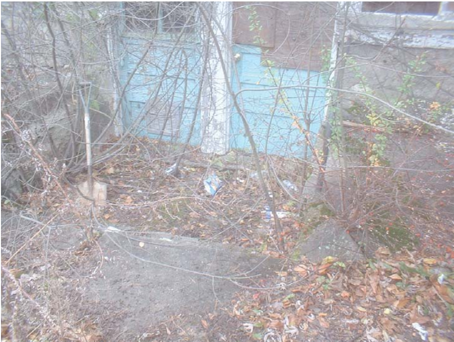
Exterior, doors to basement.
