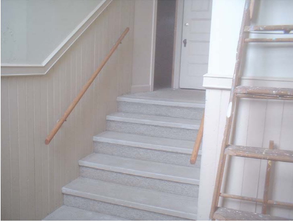
Interior, view of stairs at main entrance.
