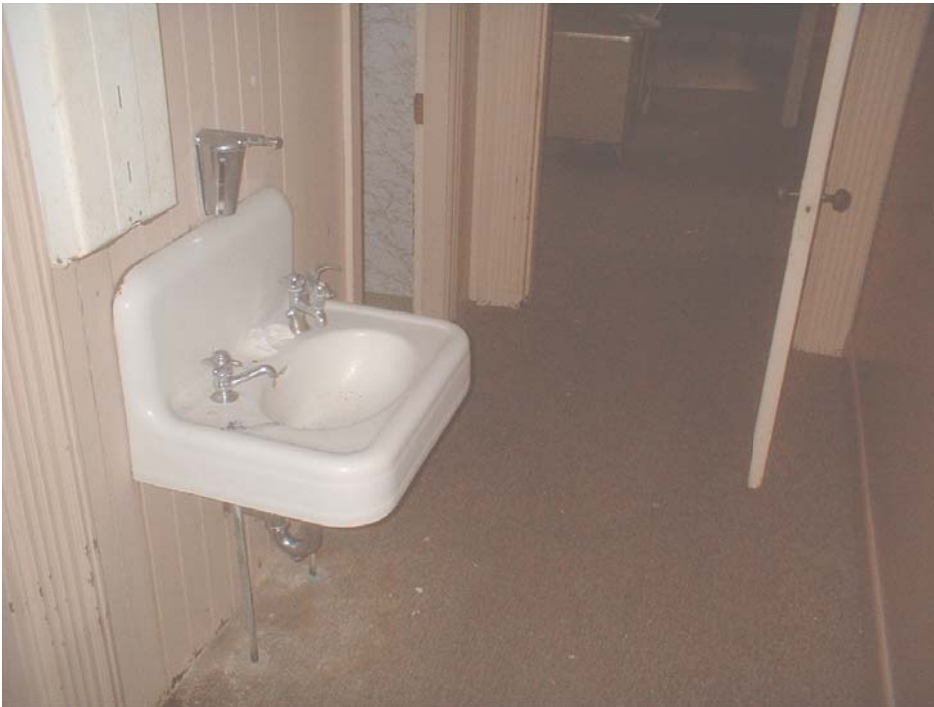
Interior, view of sink.
