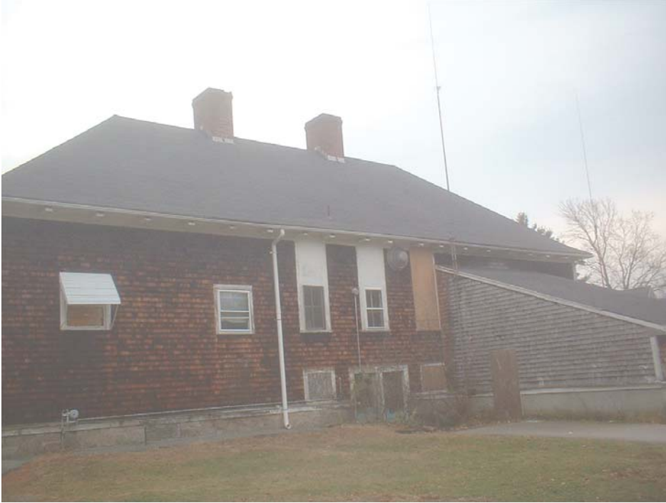
Exterior, view of back facade looking at cedar shingles.
