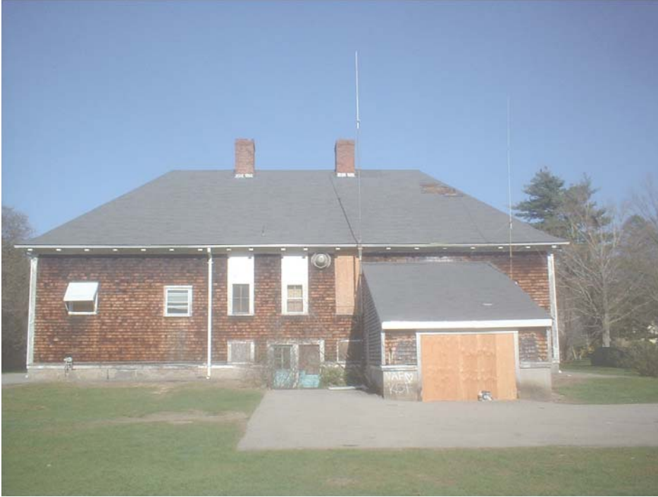
Exterior view of back facade.
